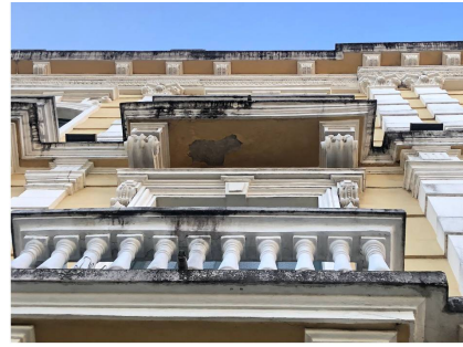
Balcão Fachada Principal
